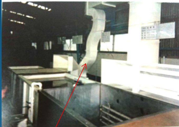
Ventilation duct
