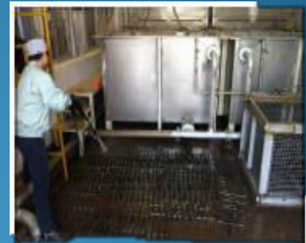
Blow away the residue of paint by high pressure water.
